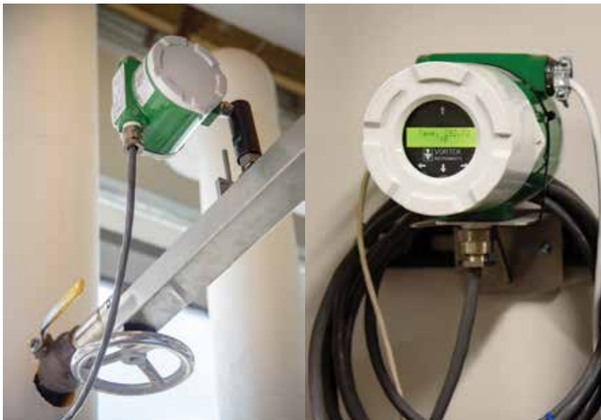
▲ Figure 4. (Left) An insertion vortex flowmeter with handwheel retractor, metering steam entering a building. (Right) Remote mounted electronics of a vortex flowmeter, metering steam. 📷 Photo by Kay Gibbs Photography, courtesy of VorTek Instruments
